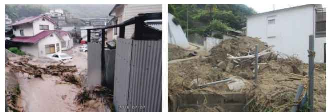
Photo 8 Debris flow hit the houses of Numata area in Hiro-Nagahama (Fig.11, No3)
