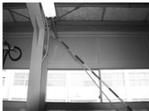
Photograph 3 Brace of Span No.13
