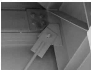
(a) Span No.15
